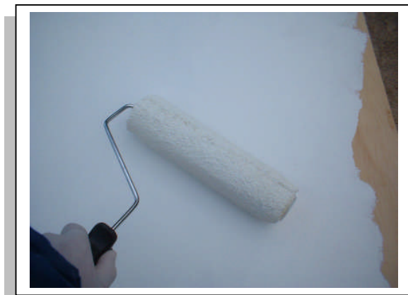
↑ Application of Everblock Stain Blocking Primer by roller
