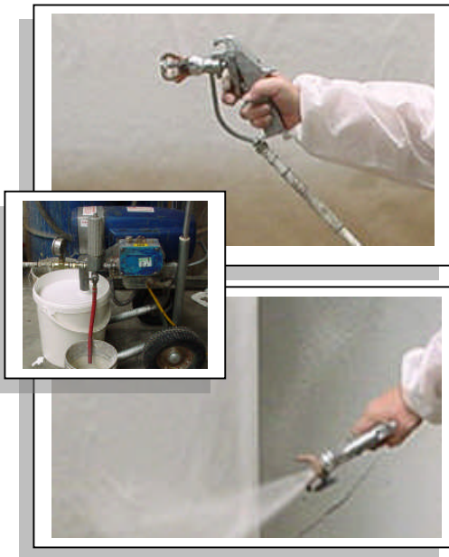
← Application of Everblock Stain Blocking Primer by airless spray
