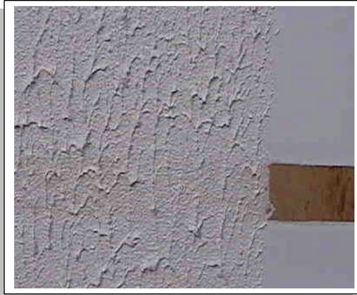
Tannin bleed through, clearly visible where Everblock Stain Blocking Primer has not been applied to the plywood background
