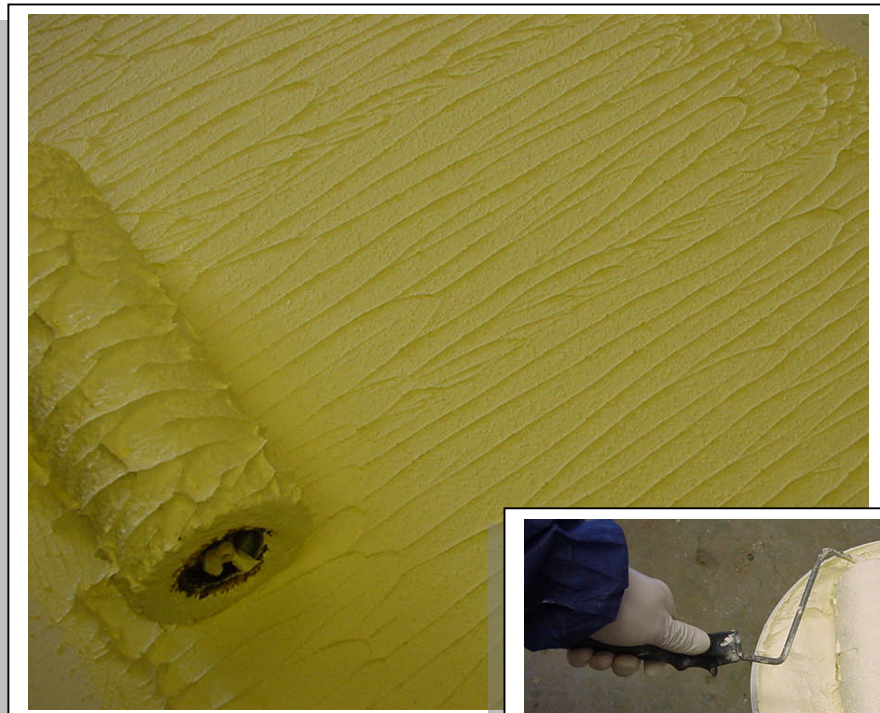
Application of Everflex HiBuild by roller
